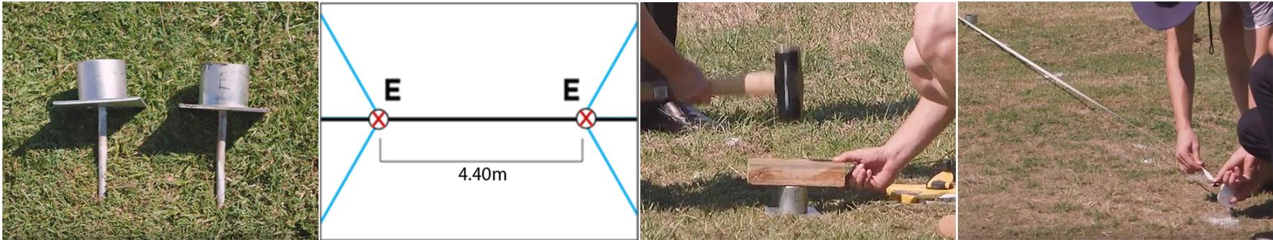
Use the supplied triangle peg placement template mark out the position of each peg. It's important that the template steps(Figure 02) to follow to identify correct peg placement, failed to follow these steps will result in your marquee not sitting in the correct position and may cause damage to the marquee.
