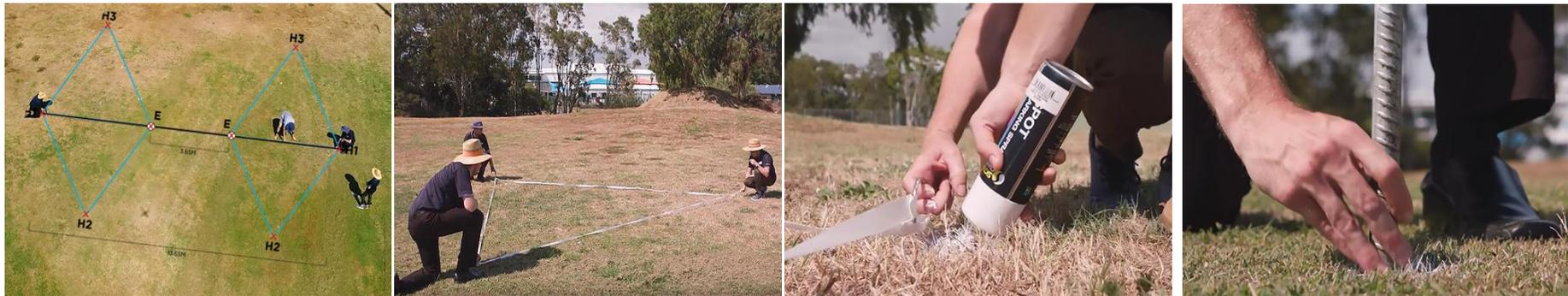
All peg locations should now be identified and drilled out in the ground using a sledge hammer, each peg must be fully drilled in the ground vertically and leaving only the top section with washers pre-drilling, they are not to be angle otherwise it will be difficult to hook the marquee legs onto them.
